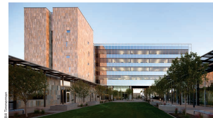
Top This water feature at the southern end of the courtyard allows water from the cooling towers to cascade down a wall into a pool. The basin is piped to the condenser water pumps.
